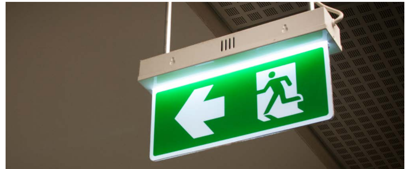
An example of an internally illuminated emergency exit sign
